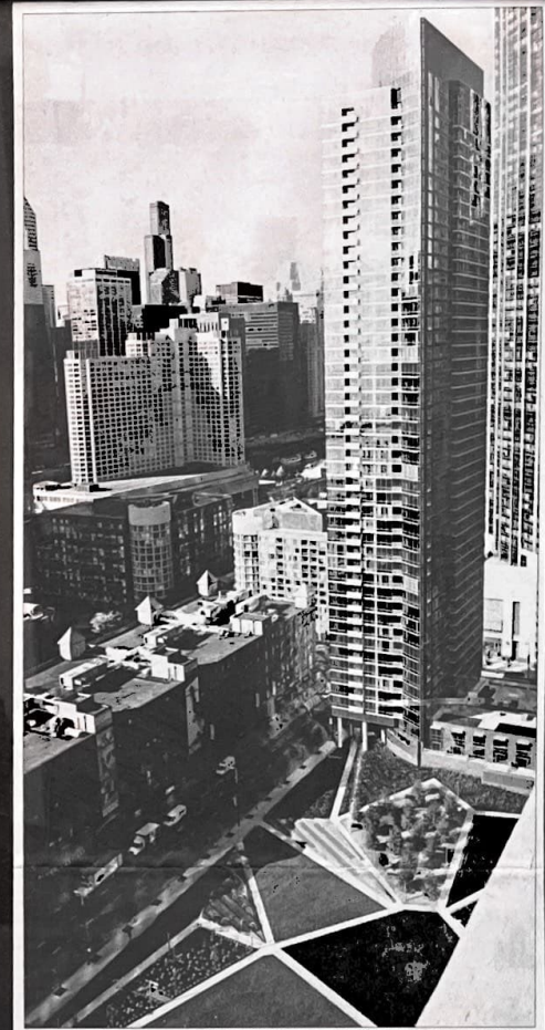
A green roof over the underground garage of ParkView Condominiums consists of sloping, mostly triangular-shaped sections that are inspired by organic. The building is faced in glass and a copper-anodized aluminum. www.parkviewchicago.com
